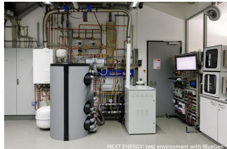
NEXT ENERGY: test environment with BlueGen
